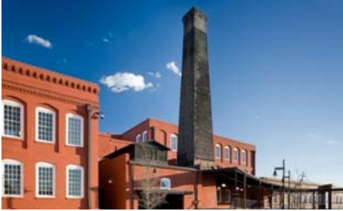
Image 4.2 The renovation of the tower - image by MNM Architects
