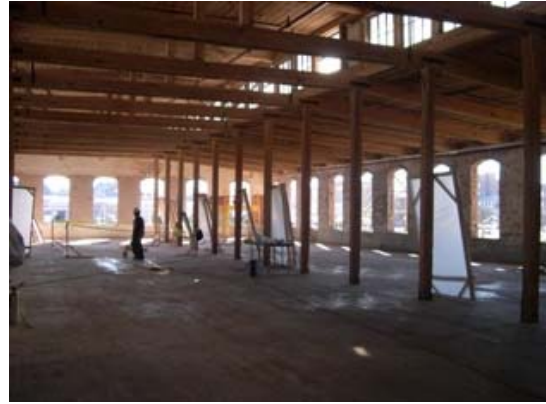
Image 3.8: Interior space of the Old Cotton Mill
