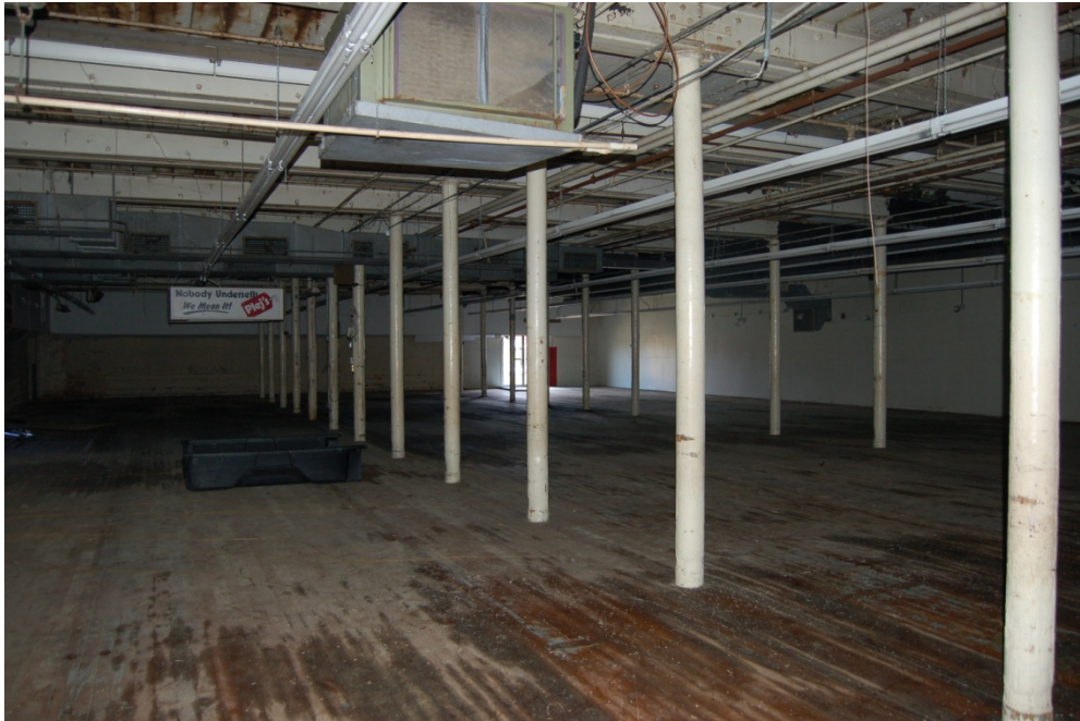
Image 3.3 Interior space of the ground floor in the addition part of the Old Cotton Mill
