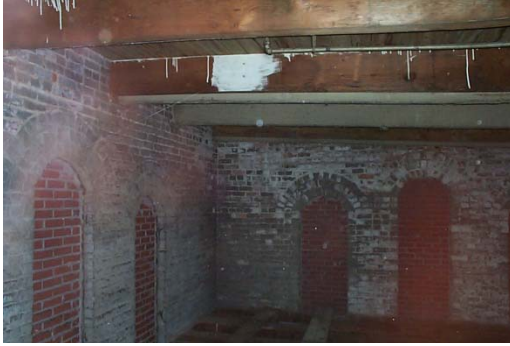
Image 3.5: View of the interior of the Old Cotton Mill
