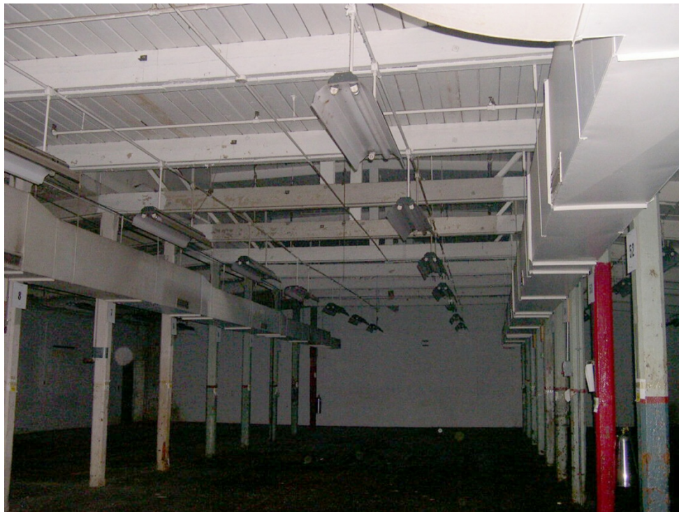
Image 3.4 Interior space of the ground floor in the addition part of the Old Cotton Mill
