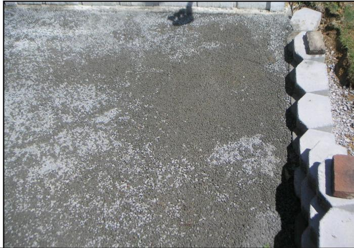
Figure 1: Example of Pervious Concrete Patio
