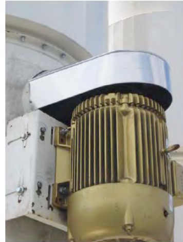
Figure 8: Fans with new cover in place
